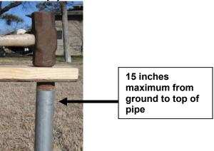
NOTE: Use a level while you are installing the pipe or Portable Mount to ensure that it is as straight as possible in the vertical plane.
