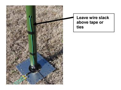
d. COMPLETELY weatherproof the vertical element wire connection and all coax feed line and unun connections using the sealant of your choice such as coax seal, silicon RTV, etc.
